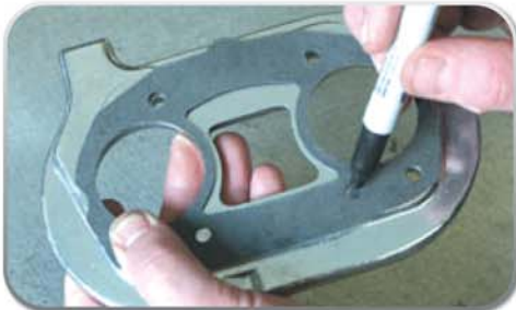
5 - Using the supplied gasket as a template, mark the center holes
